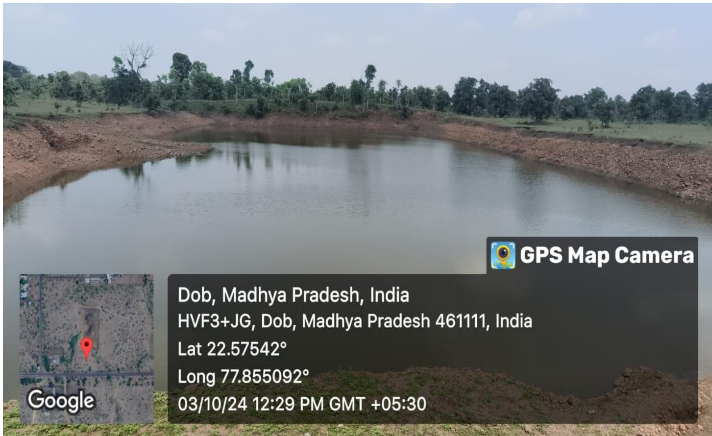
Water harvesting Pond No. 2 filled with water
